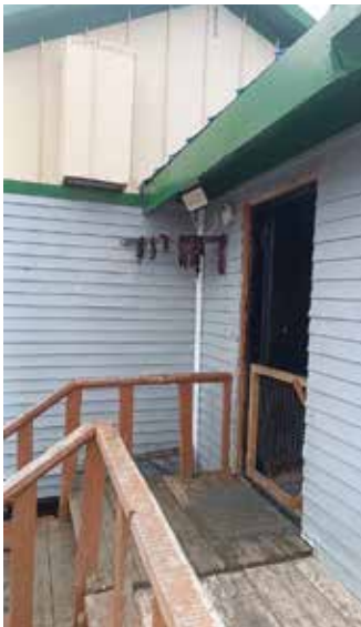
Fig. 12 Yukolniki were added to cottages facades and the dog door in Novoe Chaplino, 2024. Photo: Gavriil Malyshev.
