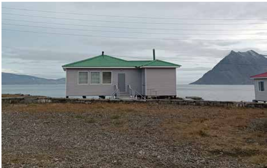
Fig. 4 Typical cottage built by Russian localization of the Canadian project in 2004 in Novoe Chaplino village, 2024. Photo: Gavriil Malyshev.
