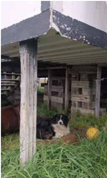
Fig. 8 Wooden blocks and wedges foundation in Uelkal, 2024. Photo: Gavriil Malyshev.
